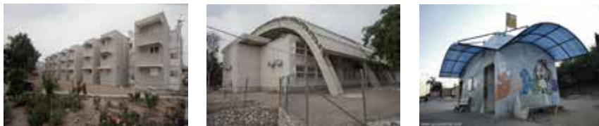
Examples for the concrete culture in the city- on the left an apartment building with added safety rooms, in the center a reinforced school building, on the right a concrete bus stop.
