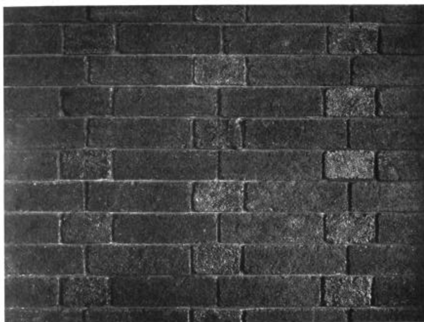
ORIENTAL METHOD OF INSERTING GLAZED TILES INTO BRICKWORK AS SHOWN IN THE INTERIOR KASCHANER GATE, KUM, PERSIA.
