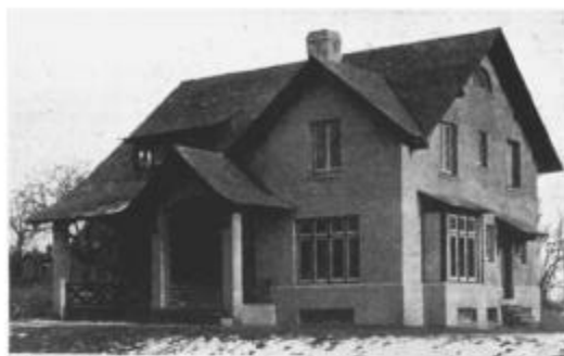
THE OUTER WALLS OF THIS HOUSE AT ALBANY, N. Y., CONSIST OF TWO 4-INCH CONCRETE WALLS WITH A 4-INCH AIR SPACE: IT WAS DESIGNED BY CHARLES R. SELKIRK, ARCHITECT, AND BUILT BY C. R. KNAPP.
