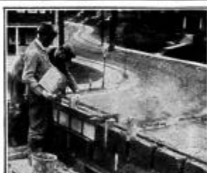
Making ready to insert the floor beams.
