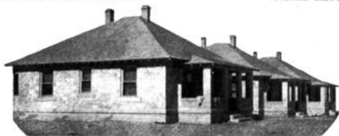
CONCRETE BLOCK COTTAGES WITH FRAME ROOFS BUILT FOR PORTLAND CEMENT PLANT EMPLOYEES IN A COLORADO TOWN AT A COST OF $1,500 EACH.
