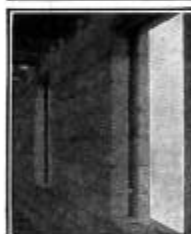
We plaster direct to the inside wall, no lathing, and stucco direct to the outside wall.
