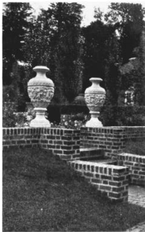
CONCRETE VASES CAST IN GLUE MOLDS FOR ORNAMENTS AT GARDEN ENTRANCE.
