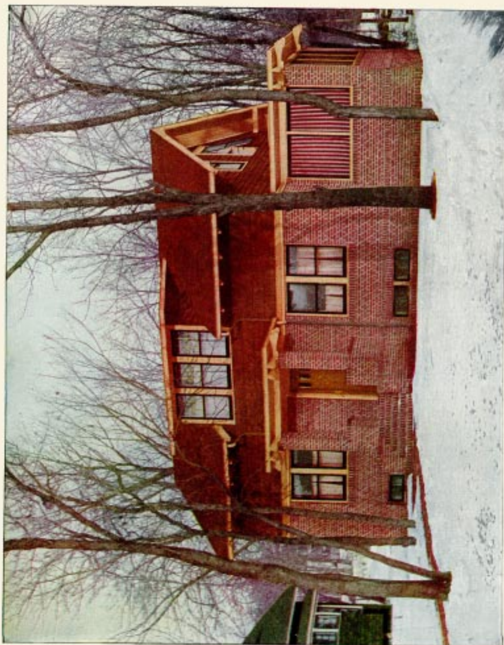
RESIDENCE, R. L. COBB, Minneapolis, Minn. Carl A. Gage, Architect. Hy-tex Colonial Brick; Dutch Cross Bond; gray mortar joint, raked one-half inch.
