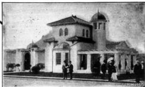
Residence of J. S. Stehlin, Long Beach, L. I. Covered with J-M Asbestos Stucco. Kirby, Pettit & Green, Architects.
