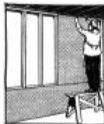
Beaver Board is nailed to the bare timbers in new buildings or over lath and plaster in old buildings.
