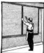
After Beaver Board has been painted, the decorative strips are nailed over the edges, giving the beautiful modern panel effect.
