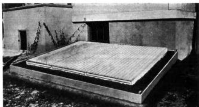
SAME FRAME ENCLOSED IN A SUBFRAME, THE MOATLIKE SPACE FILLED IN WITH LEAVES AND LITTER, AND THE GLASS COVERED WITH SHUTTERS FOR WINTER WARMTH.
