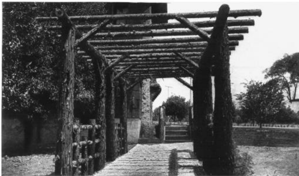
A PERGOLA SHOWING THE CHARM OF A COMPLETELY RUSTIC EFFECT: OLD TREES HAVE BEEN TRIMMED FOR THE SUPPORTS AND RUSTIC BRANCHES FORM THE ROOF: THE DRAPING OF GRAPE-VINES GIVES JUST THE INFORMAL FINISH NECESSARY. RUSTIC PERGOLA CONSTRUCTED ENTIRELY OF CALIFORNIA REDWOOD LOGS AND POLES: THE WALK IS OF GRAVEL: THE VINE COVER FOR SUCH A PERGOLA WOULD SEEM TO BE CALIFORNIA ROSES.
