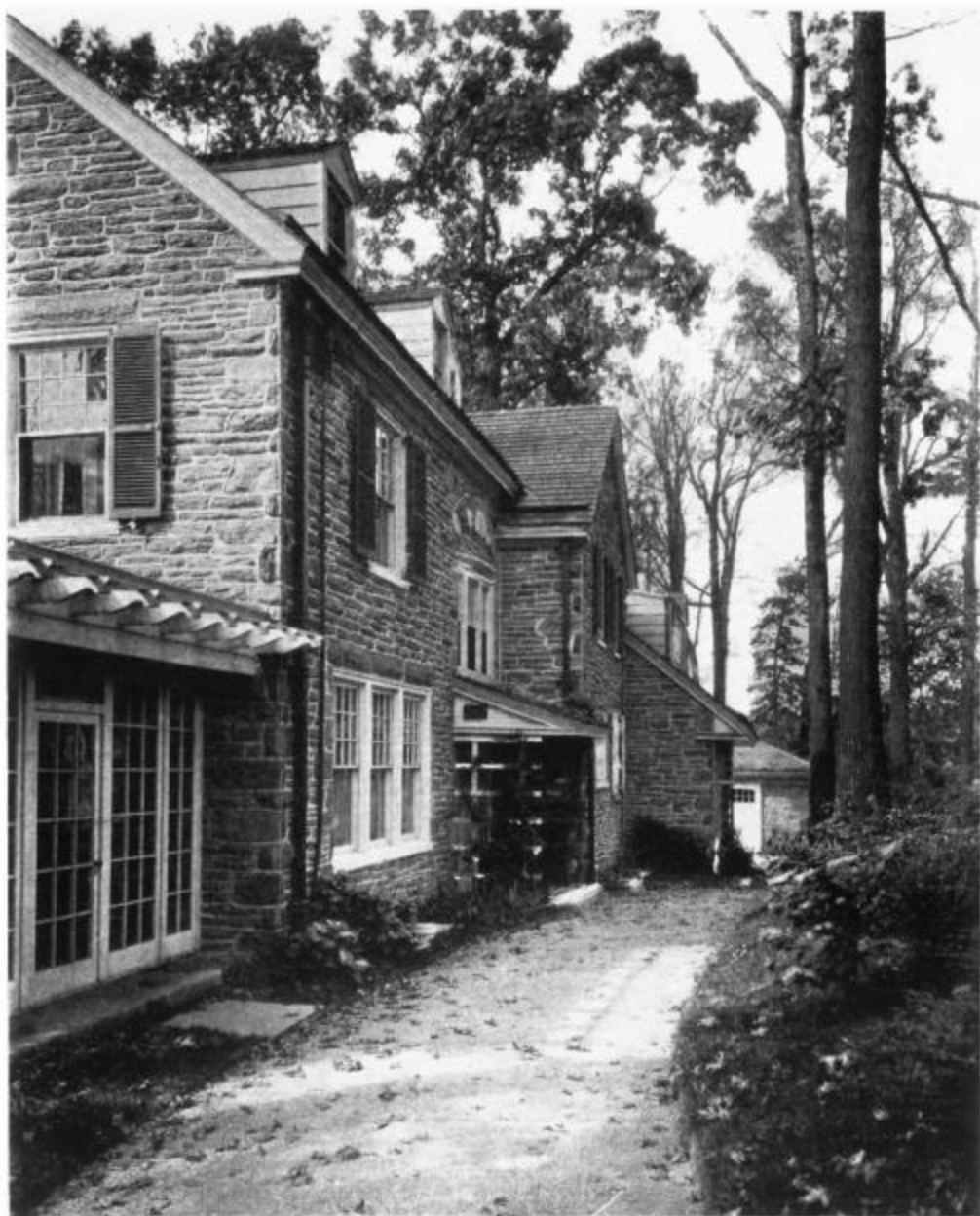
TERRACE at the back of the Harry T. Saunders house showing in detail the effectiveness of the Germantown type of stone laying.
