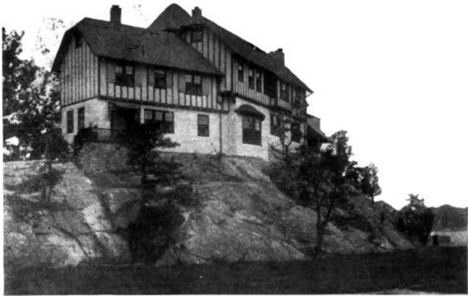
ROMANTIC SUMMER HOME built at Tokeneke, Connecticut, upon a narrow ledge: The large tower that runs through the center of the house was cut out of the solid rock.
