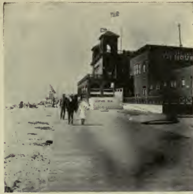
Am Eng. Co. SECTION OF THE LONG WALK. Photo. by Engelbrecht
