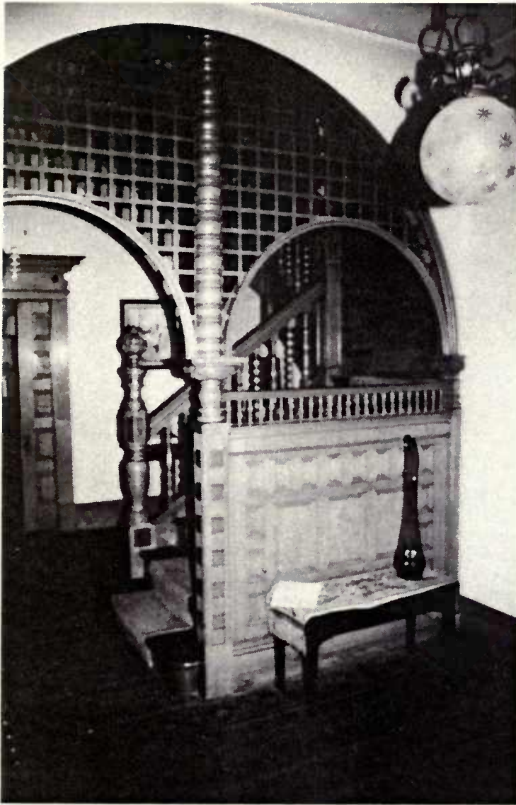
Left: Entry hall of restored G. W. Patterson house
