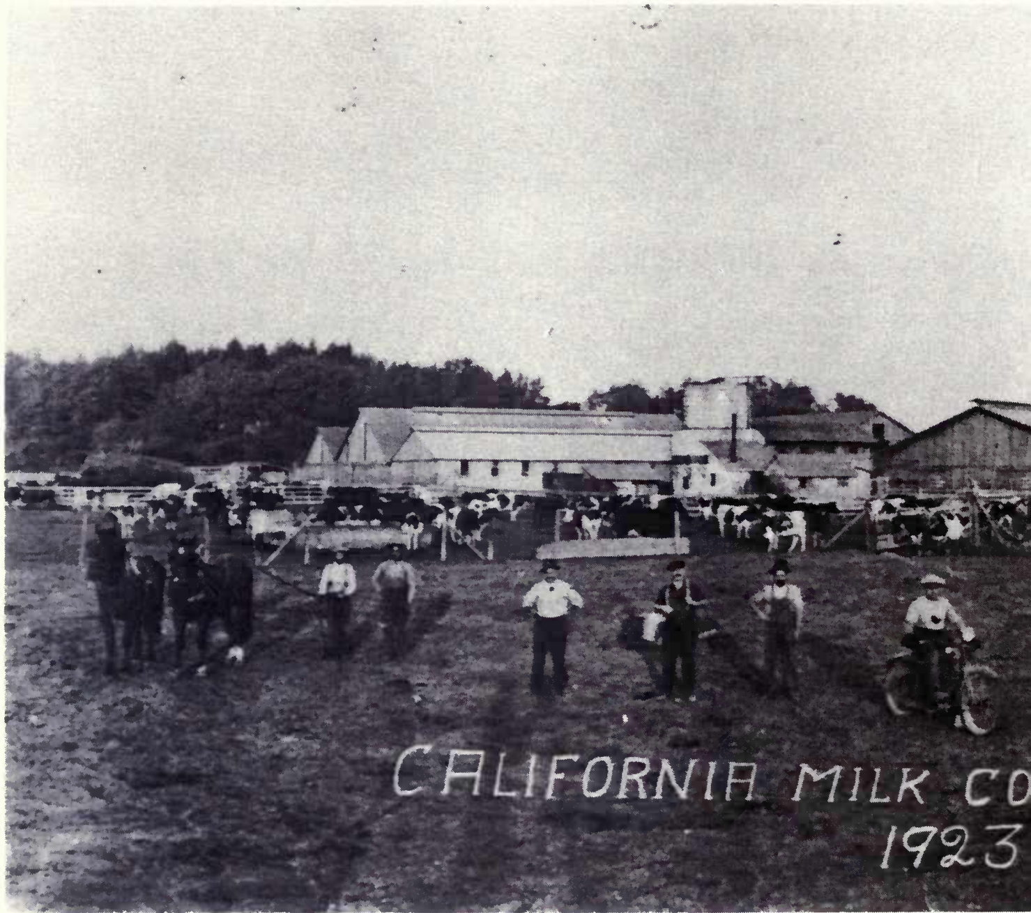
Dairy on Patterson Ranch, managed by Fran
