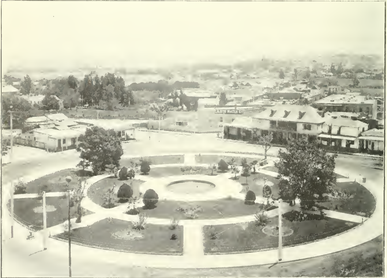
The Plaza, Looking Northeast. The Old Spanish Buildings Are Being Torn Down to Give Space for the New Warehouse District.
