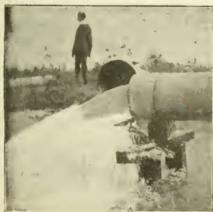
One of Our 12-inch Wells
