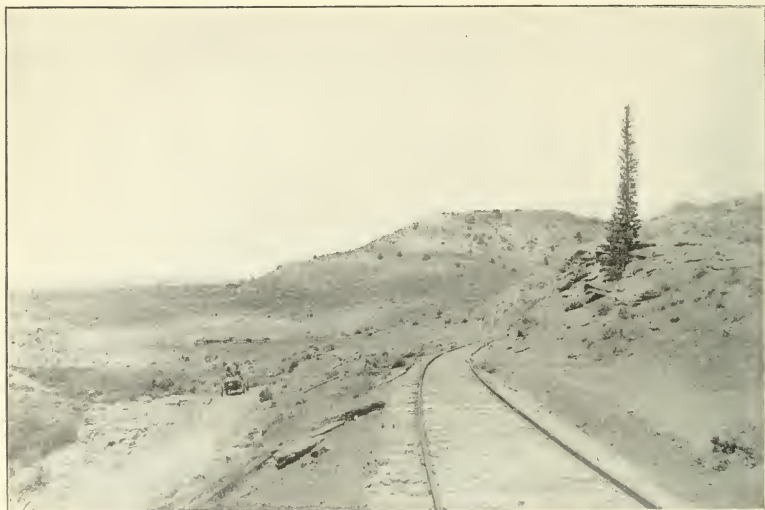
Often the Road Parallels the Railway.
