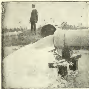
One of Our 12-inch Wells
