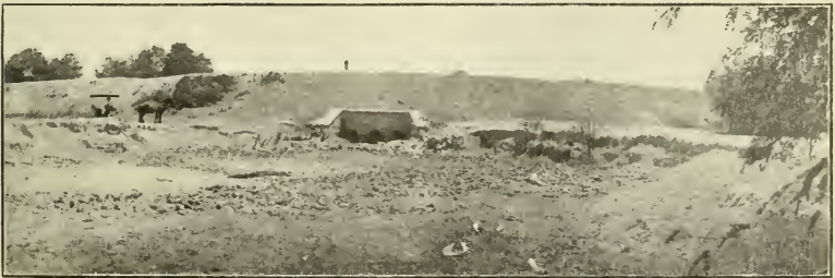
Bank of Great Reservoir, Showing Intake for Lower Canal.
