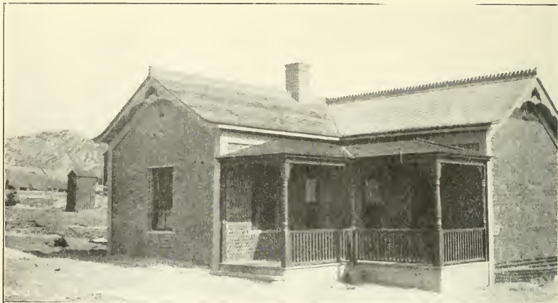
Cottage Built of Bottles and Adobe, Bullfrog District; 40,000 Bottles Are Embedded in the Walls.
