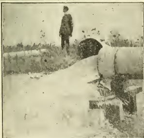
One of Our 12-inch Wells
