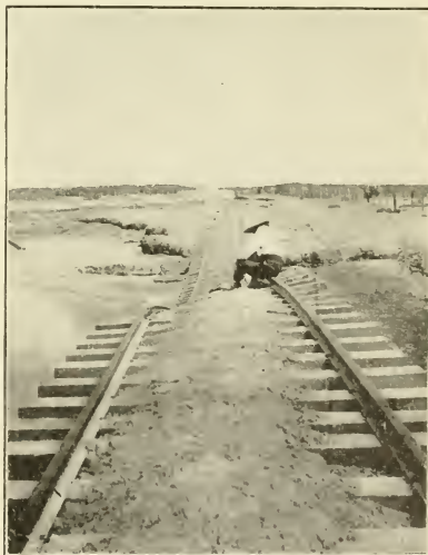
Head of Overflow in New River Near Packard, Mexico.
