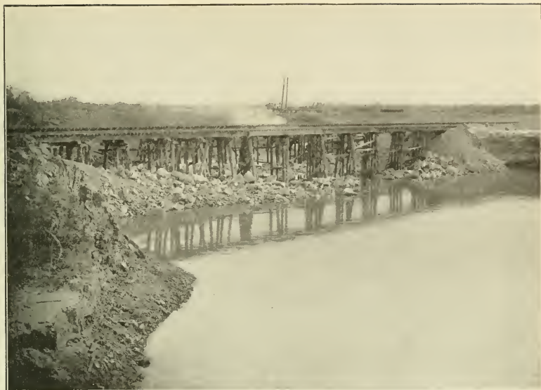
Closure of the Gap Made by the Failure of the Rockwood Gate.
