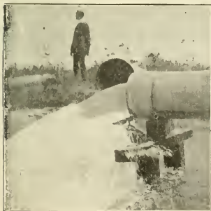
One of Our 12-inch Wells
