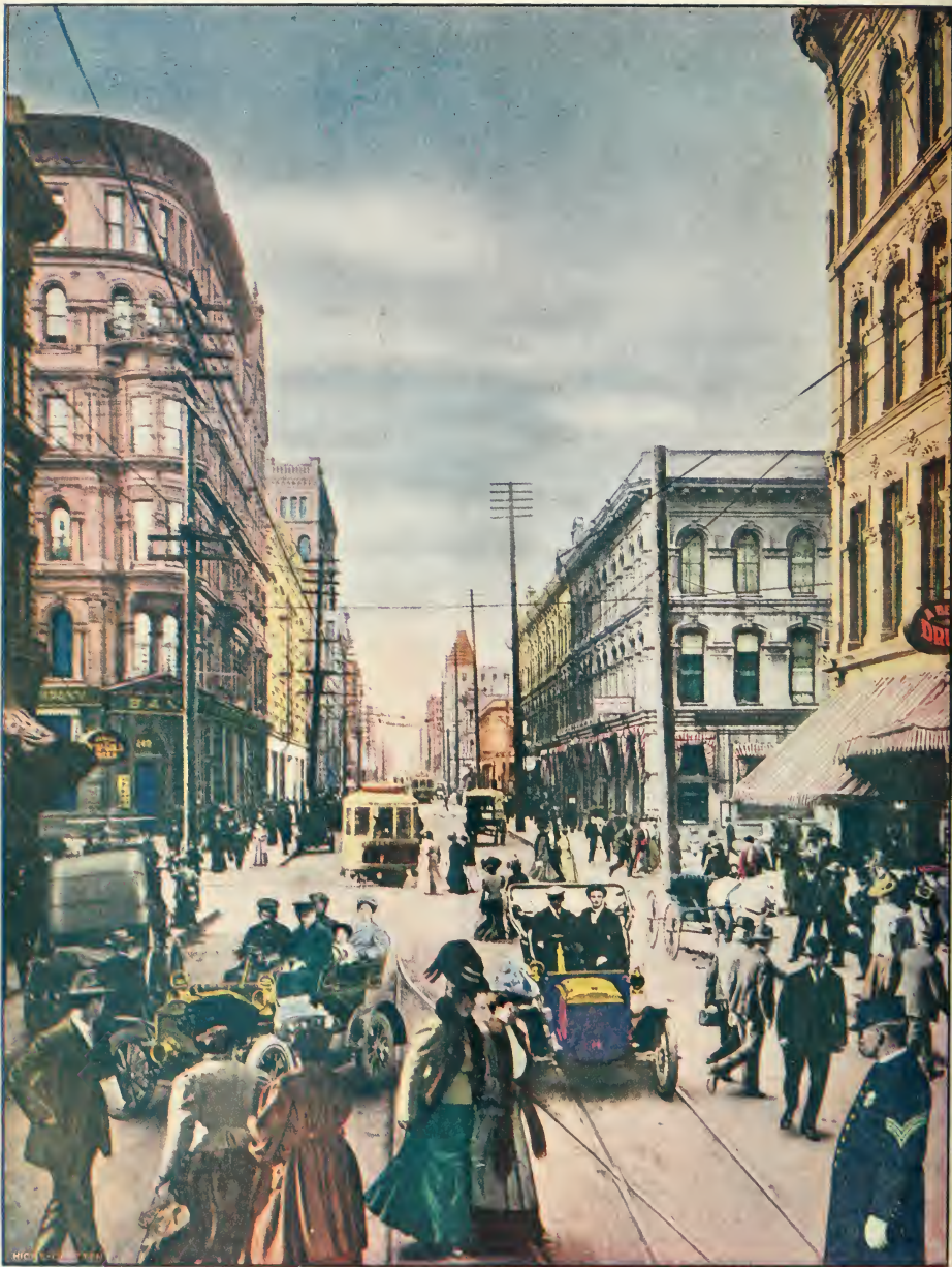
Washington Street, Portland, Oregon, paved with wooden blocks preserved with AVENARIUS CARBOLINEUM.
