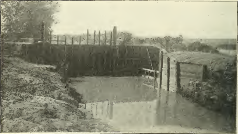
Headgate of Casa Grande Valley Canal—Gila River at the Right.
