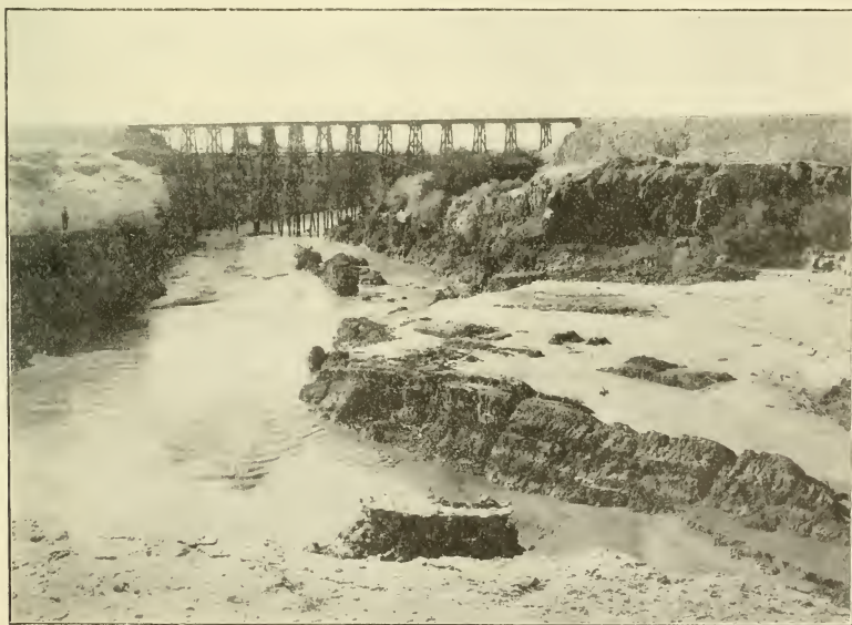
The Alamo River, a Channel Just Above the Holtville Railroad Bridge, Showing the Cut Channel Which Almost Washed the Bridge Out.
