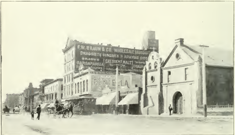
The Old Mission Church Flanked by "Gringo" Business Structures.
