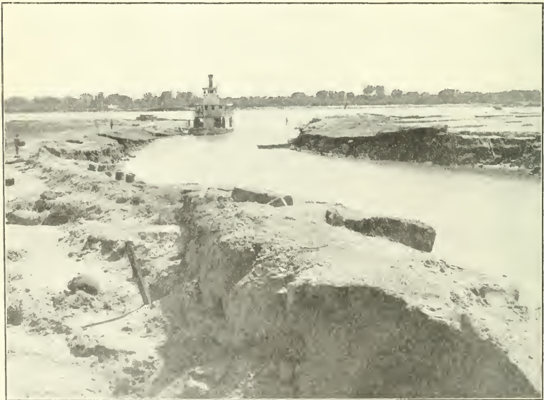
Looking Out Toward the Main Channel of the Colorado River, Showing the Steamboat Standing at the Entrance of the Diverting Channel, at the Headworks of the California Development Company's Dam in the Colorado River, Just Below the Old River Bed.
