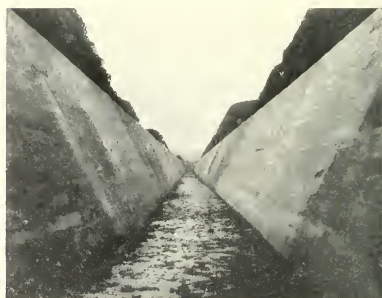
Ditch Lined With Concrete to Carry an Entire River—the Truckee.
