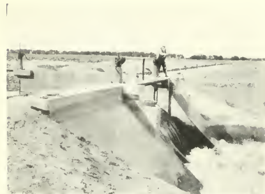
Waste Hole on One of the Main Laterals.
