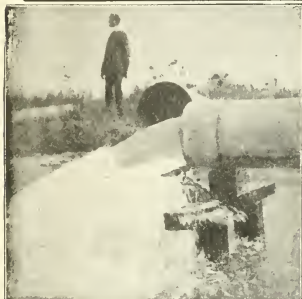
One of Our 12-inch Wells
