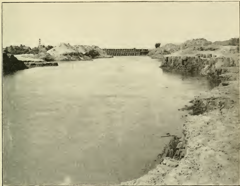
Looking Down the Proposed Diverting Channel at the Headworks of the California Development Company's Dam, Showing the Channel Which Is Supposed to Carry the Water in the Colorado River Around the Works While the Dam Is Being Built. The Rockwood Gate Before It Went Out.
